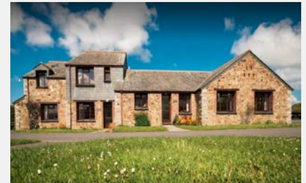
1MWh Olde House Project in Cornwall supported by Centrica
